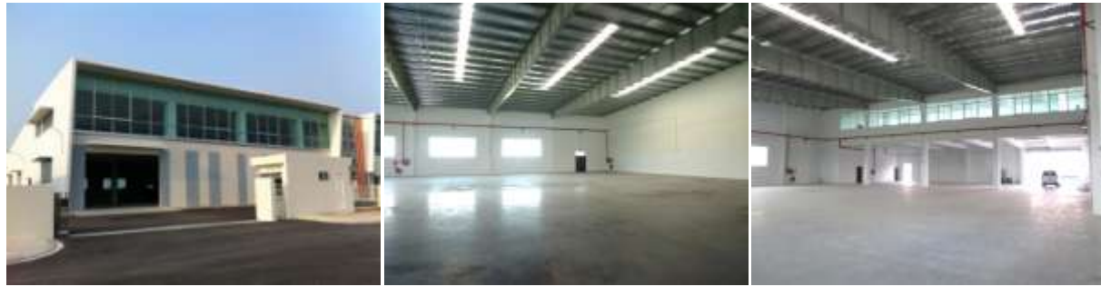
RBBS2000 factories: 2,000sqm of column-free production and floor-to-ceiling glass windows at mezzanine office
