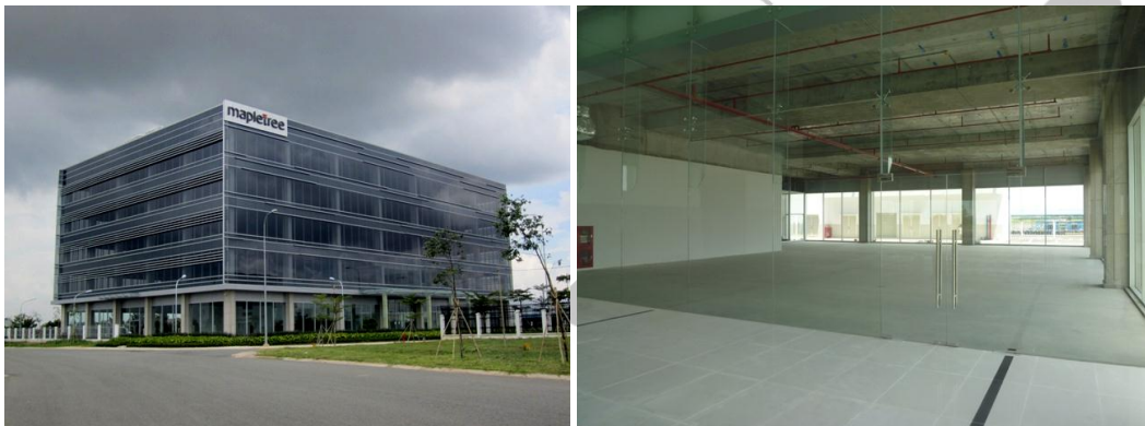
Completed 5-storey office building – 2,000sqm column-free office space per floorplate
