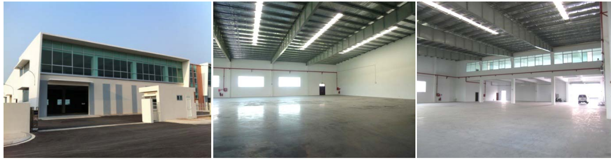
RBBS2000 factories: 2,000sqm of column-free production and floor-to-ceiling glass windows at mezzanine office
